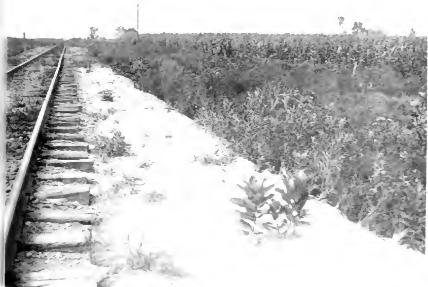
Fig. 1. Station I. Looking northeast over the north portion of the station.
